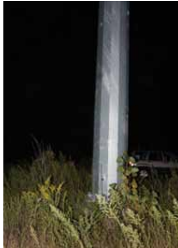
The power pole
