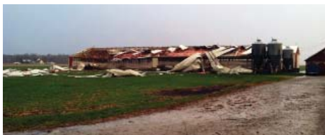
Storm Damage on Barkley Road Near S.R. 101 (south of Monroeville)
