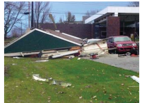
Storm Damage in New Haven, Indiana
