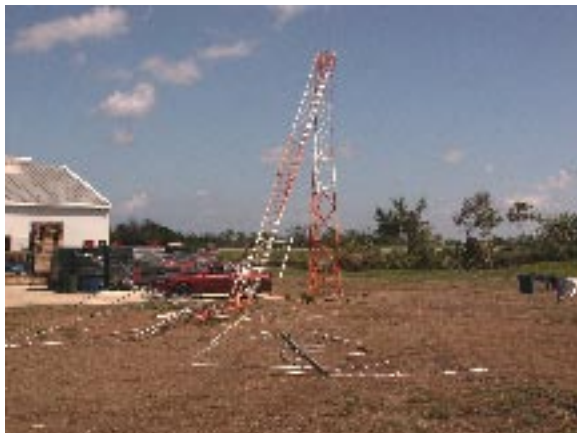
Fig 1 The 'old' main tower right after Hurricane Ivan
