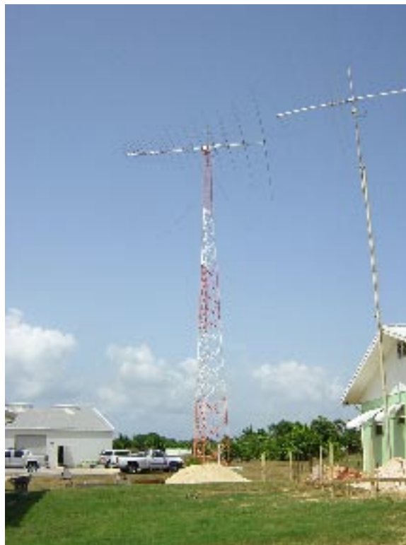
Fig 2 The 'new' main tower, with the 40-10 m log periodic array at 100 ft (that's a C3 on the right).
